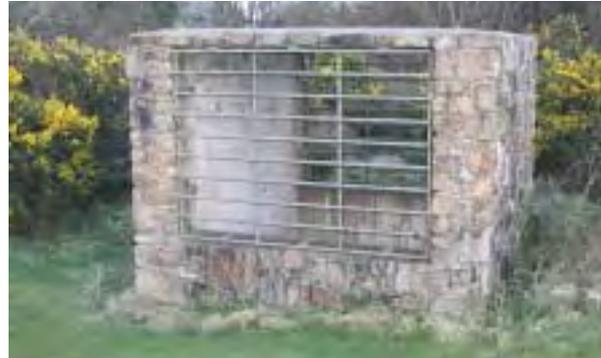
Mine shaft safety enclosure at Tresavean Mine, Lanner, designed to permit access for bats which roost in the underground workings. Measures to make provision for protected species such as bats, barn owls and badgers, should be carried out in sympathy with the historic environment.
